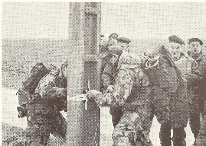
Preparing the concrete pylon for the 'off'.
